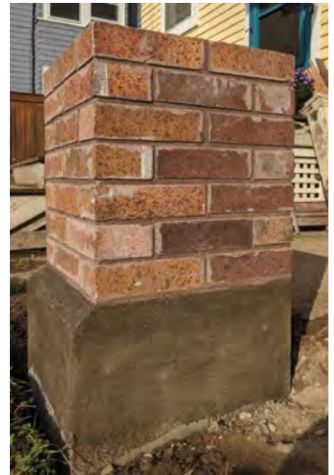
Newly reconstructed piers with our original brick and similar salvaged brick. Can you spot the difference?
