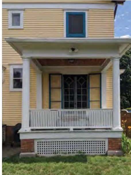
Back porch of the subject property. The brick pier on the left of the image is sinking most noticeably.
