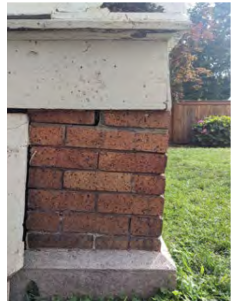
Closeup of sinking brick pier. Note the brick at the top that has shifted.
