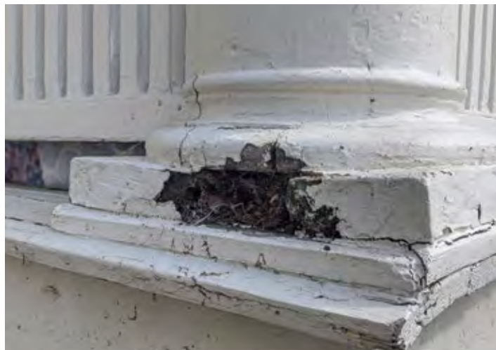
Column base that has rotted over time.
