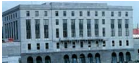
Rundel Memorial Building
