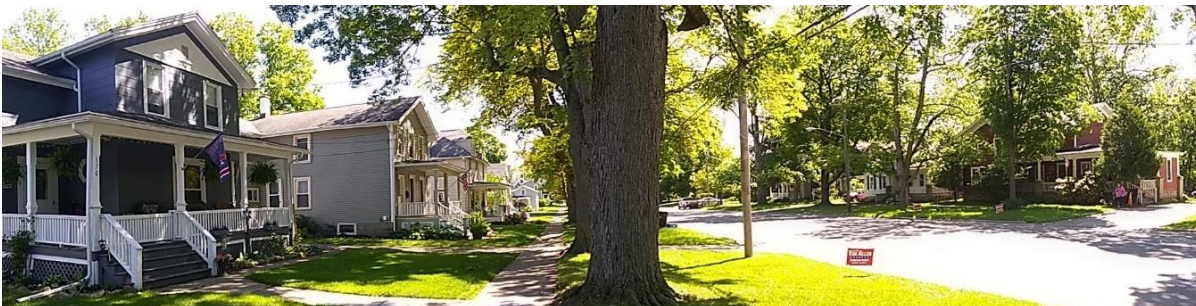
Figure 19a. view southward along Genesee St. from near intersection w/ Clinton. Note modest scaling, later styling compared to houses on E. Main St., but common setback & massing unites area
