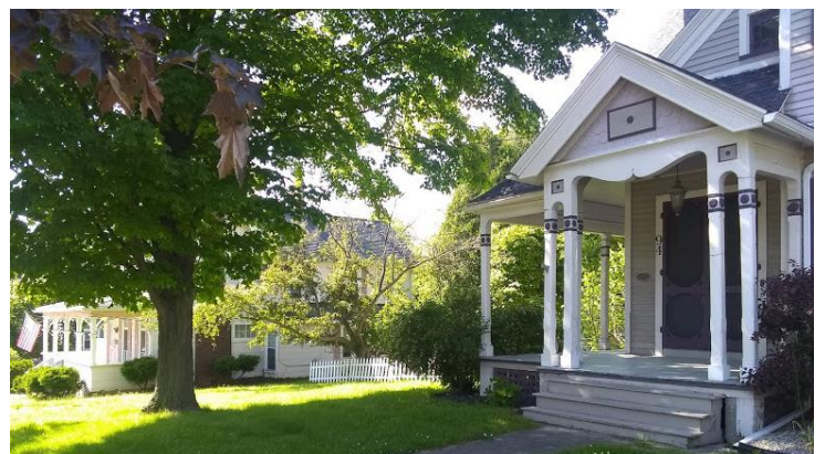
Figure 20. Detail of 86, 94 E. Main, exemplifying unifying decorative woodwork
