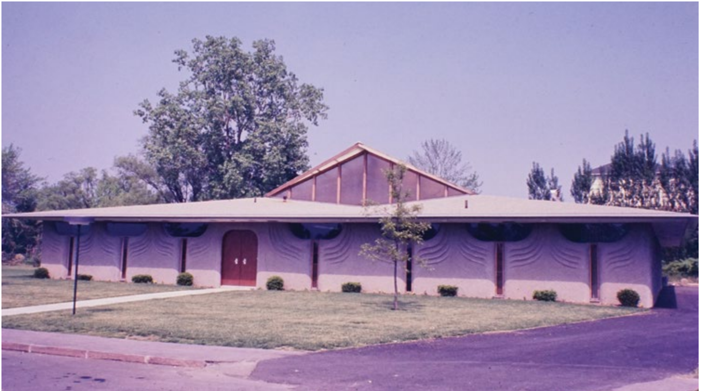
Our Lady of Mercy Rectory, Greece (1965). This was Johnson's first earth-formed concrete building, using a process he developed with ceramic artists James and Philip Secrest. It is also the only one of his six earth-formed concrete buildings that has been demolished. Historic view from the James Johnson Slide Collection.
