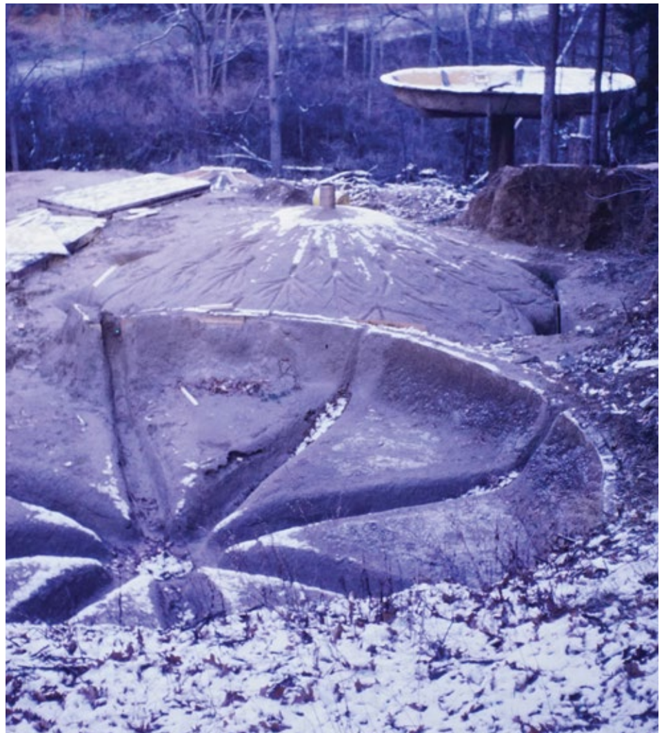
Antell-Whitman House, Perinton (1969). The "Mushroom House" pods were built using two molds created at the site, one for the upper halves and one for the lower halves. This photo shows the two molds (foreground and middle ground), with the building under construction in the background. James Johnson Slide Collection.
