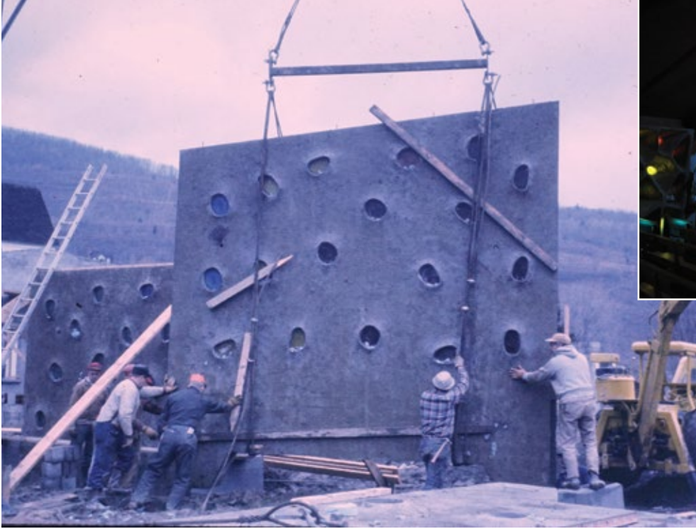
St. Januarius Church, Naples (1965-66). This construction photo shows the concrete panels that form the exterior walls being tipped into place, having been formed on site in a mold created in the earth. James Johnson Slide Collection.
