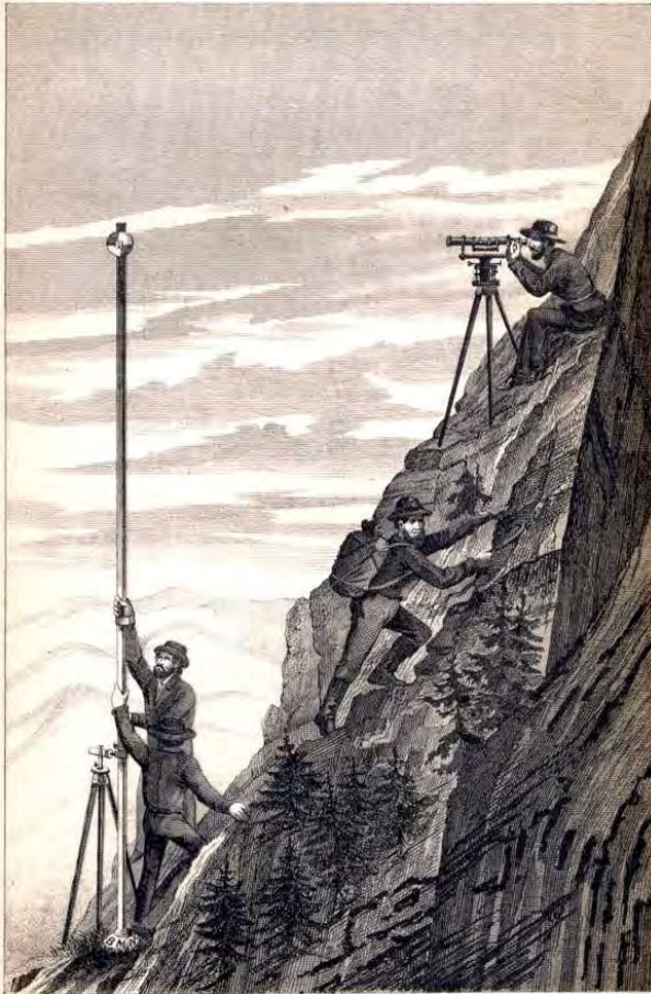
DIVISION OF LEVELS. Measurement of Whiteface Mountain, with Spirit-Level and graduated Rod
