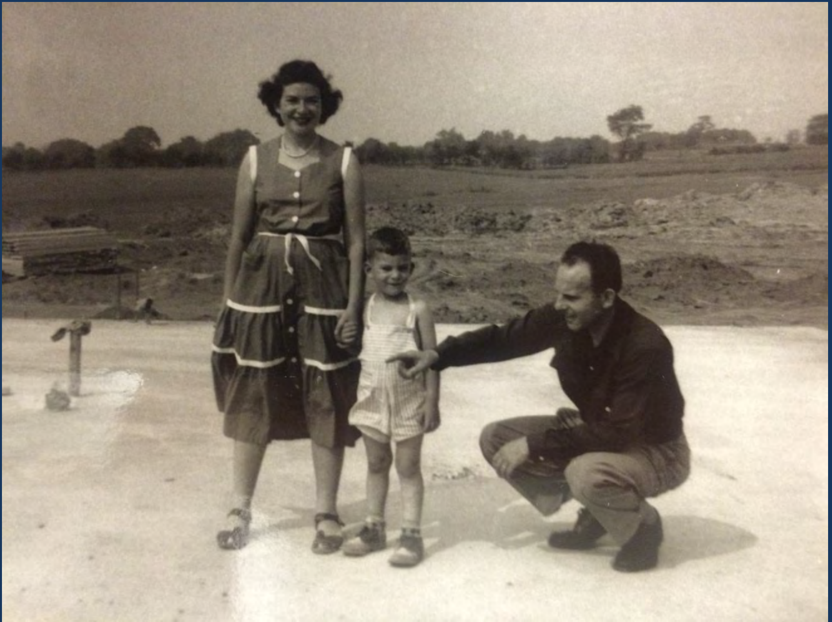
Elsie, Ira, and David Freedman on concrete pad for their house at 46 Bailey Ave
