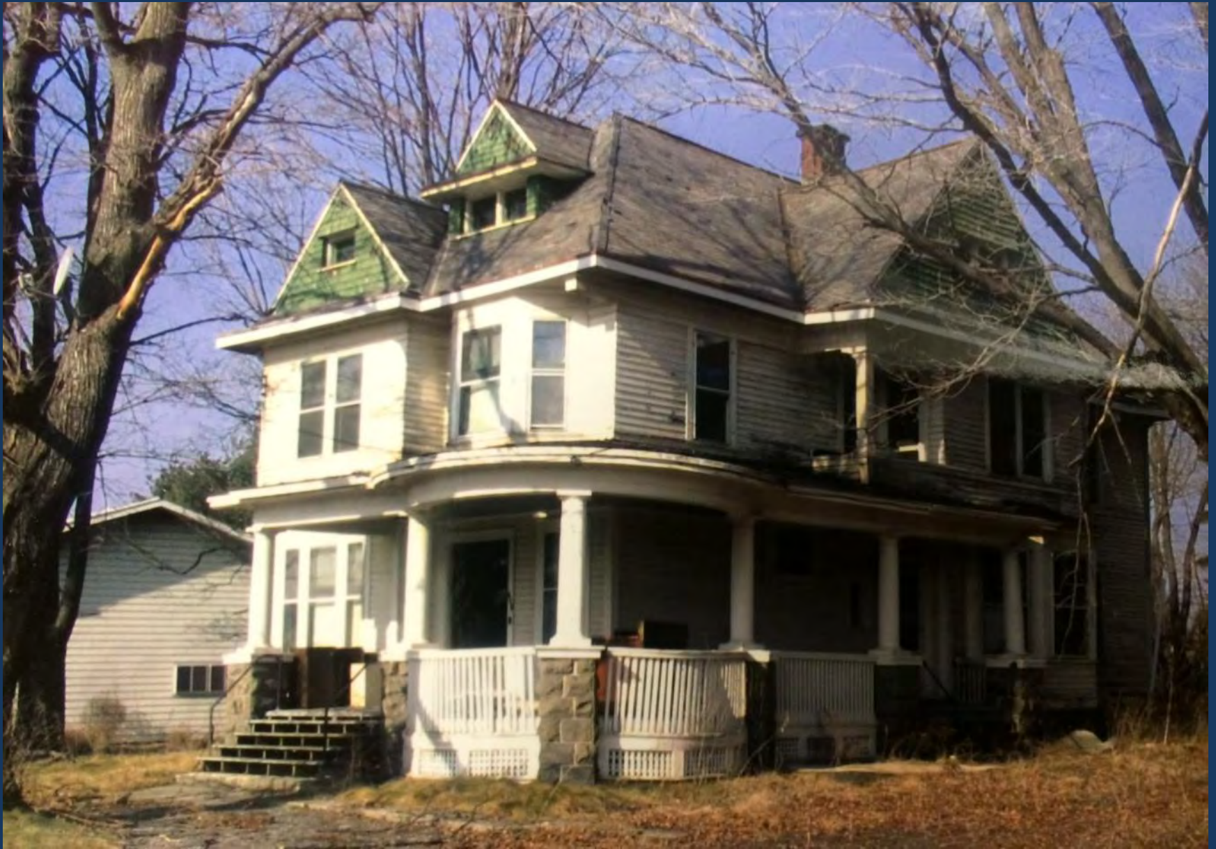
Former Burns-Whitney Farmhouse (demolished)
