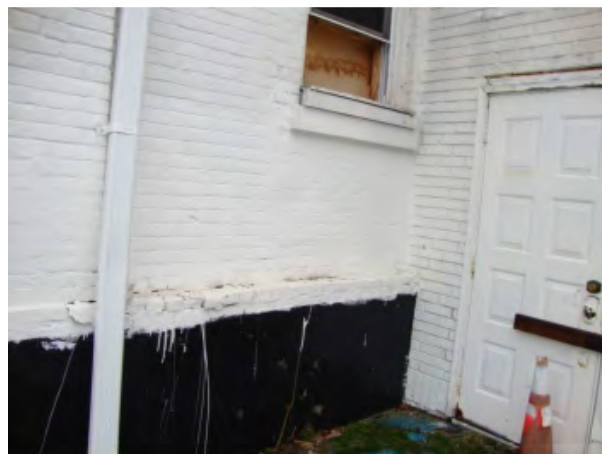
Image 12- East Entry Door
