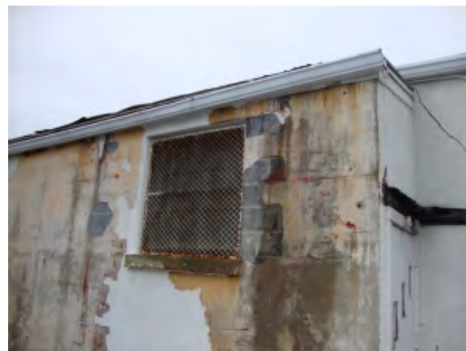
Image 14- Stucco damage
