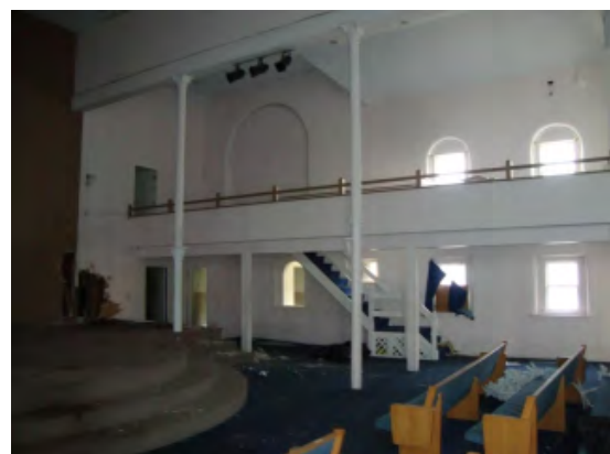
Image 04- Sanctuary NE Mezzanine
