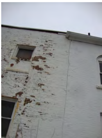
Image 11- East Entry Brick Joint
