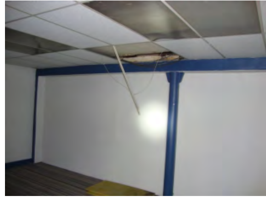
Image 06- First Floor Space
